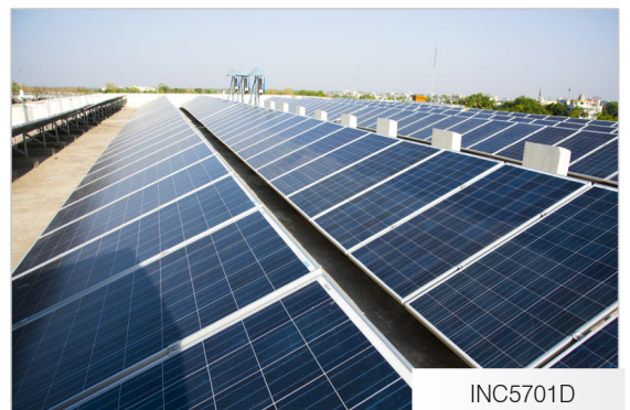
Alignment of solar and photovoltaic panels
